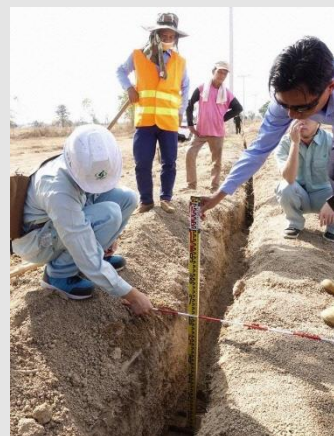
▲ JICA Grass-roots technical cooperation (Coaching for method of pipe installation)
